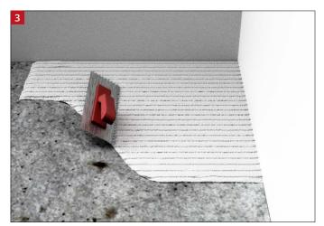
Ultralight should be installed using a flexible, cement-based adhesive. The adhesive should be trowelled out and combed through using a 6 mm x 6 mm ( $\frac{1}{2}$ " x  $\frac{1}{2}$ ") square notch trowel to give a ribbed bed, any slight depressions in the subfloor being filled by the mortar.
