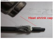
**4.** Pull the pushed-back braid over the sealed end cap and twist the braid end together.
