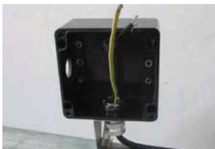
**18.** Make connections as shown in the following figures. Connect the power wires with the cable wires. Connect the incoming ground wire with the cable braid. The wire nuts, included, must not be connected with aluminum wires. The junction box also needs to be grounded.
