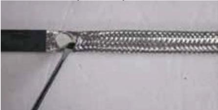
4. The heating cable must be bent so the insulation can be pushed out of the braid.
