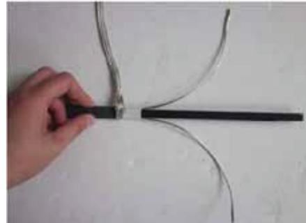
8. Cut off remaining PTC material, leaving the exposed wires. **Do not cut bus wires!**
